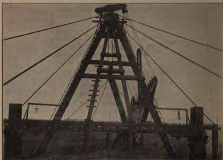
A-frame of Floating Dipper Dredge. Figure 81.
